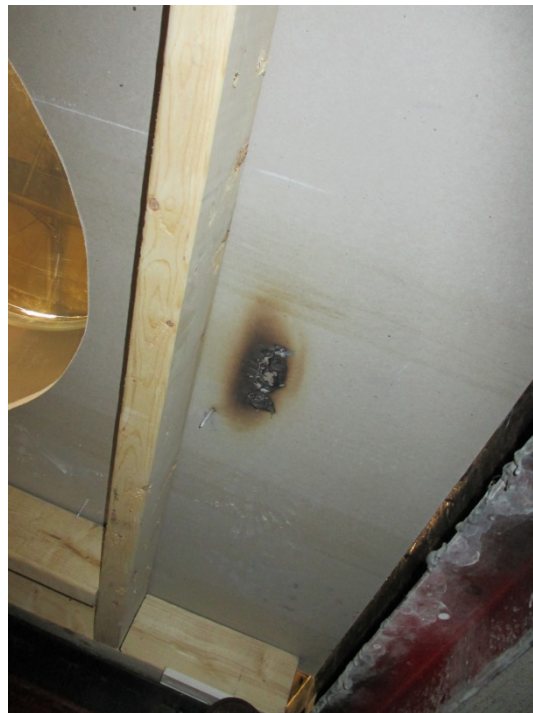
Photo No. 6 Underside of Gypsum Board (During Test)
